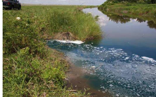
Photo 1 (Upper Left). Five thousand gallon water truck used to treat part of the subsurface drainage system. Photo 2 (Upper Right). The water hose from the tank truck used to apply rotenone to the subsurface drainage system. Photo 3 (Lower Left). Water tank truck used to treat subsurface drainage system. Photo 4 (Lower Right). Blue dye used to indicate when the full length of the subsurface drainage pipes had been treated.
