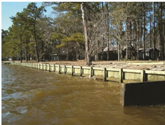
Figure 5.19. Bulkhead designed to control wind-induced shore erosion. Photo credit: M&M Marine Construction, Queenstown, Maryland.
