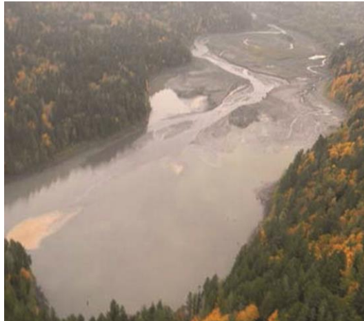
Figure 3.16. The sediment built up in the upper end of Lake Aldwell, impounded by the Elwha Dam, Washington, was exposed by a drawdown, eroded by the river, and flushed downstream. The dam was eventually removed, and the Elwha River flowed freely through the site by March 2012. Photo credit: B. Cluer.
