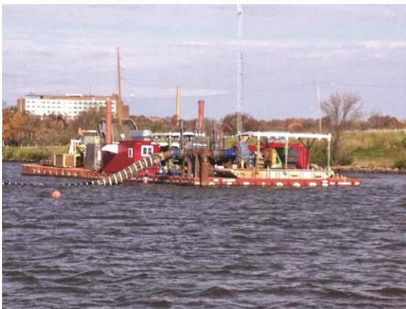
Figure 3.12. Hydraulic dredging at Decatur Lake, Illinois, part of a $91 million reservoir restoration. Photo credit: M. Honnold, Macon County, Illinois.
