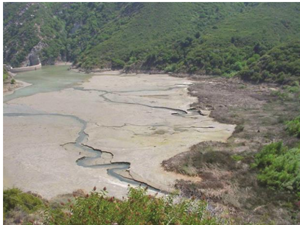
Figure 3.1. Matilija Dam, on the Ventura River Basin, California, was constructed in 1947 and is nearly completely filled with sediment. When constructed, the dam was 190 ft high and impounded a volume of 7,000 ac-ft; by 2015 it was reduced to 400 ac-ft. Photo credit: P. Jenkin.
