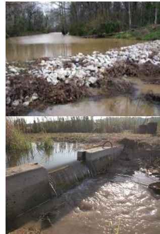
Figure 9.6. Weirs installed to retain water and prevent premature dewatering of backwater areas. Photo credit: USACE, Rock Island District (upper), and R. Kröger, Mississippi State University (lower).
