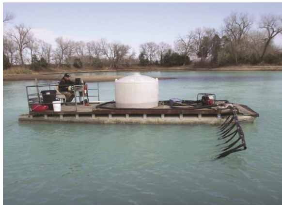
Figure 4.6. Applying alum at a Nebraska reservoir. Photo credit: M. Porath, Nebraska Game and Parks Commission, Lincoln.
