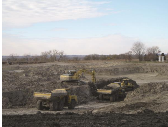
Figure 3.10. Excavation of accumulated sediment at a Nebraska reservoir. Photo credit: M. Porath, Nebraska Game and Parks Commission, Lincoln.
